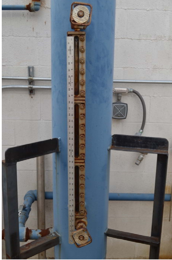
Water Storage Tank
